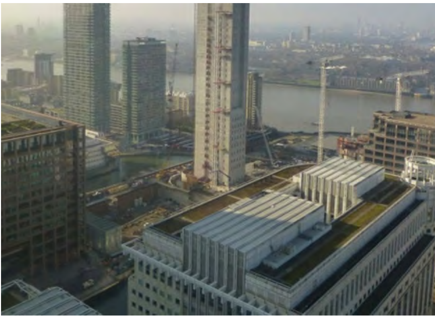
Massive Isle of Dogs developments causing strain on mains utilities. Picture source: Isle of Dogs Forum
