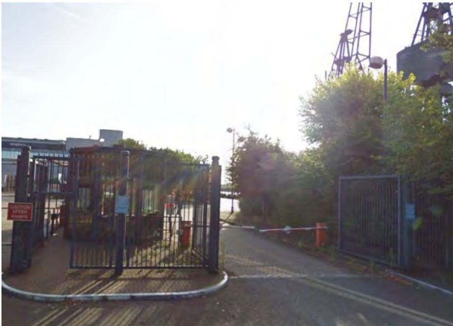
Entrance to Westferry printworks site on Isle of Dogs after being flattened for redevelopment. Picture source: Google
