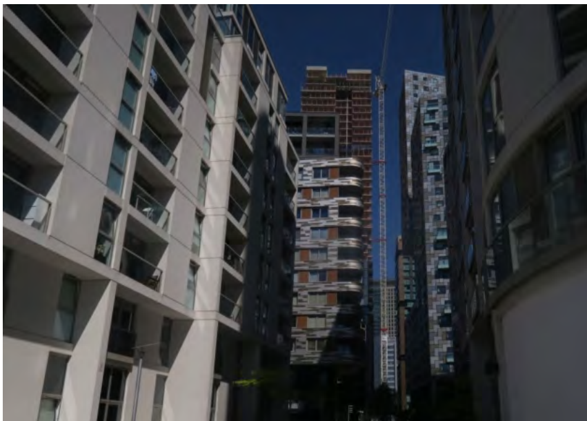
Massive housing development on the Isle of Dogs with yet more construction going ahead. Picture: Mike Brooke
